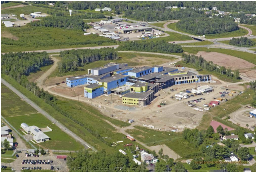
Figure 1 Truro:::Colchester's new hospital near hwy 102 is now nearing completion
